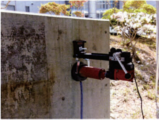
Fig.5 Sampling of concrete core
