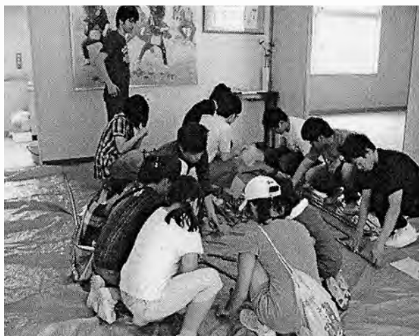
Fig.5 Scene of the joint work for assembling aeration tube placed in the pond water of Kashiko-numa Pond at Taira-Numanouchi community center. (27-Jun-2009)
